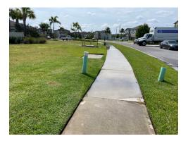
Item 10Sidewalk repair is needed where water is pooling.
