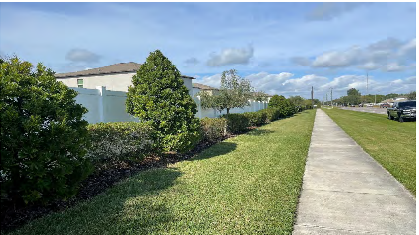
The landscape along 78 th street is in good condition.
