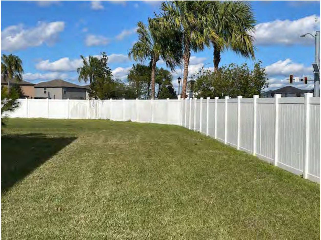
The fence has been repaired at the end of Ginger Lily Ct.
