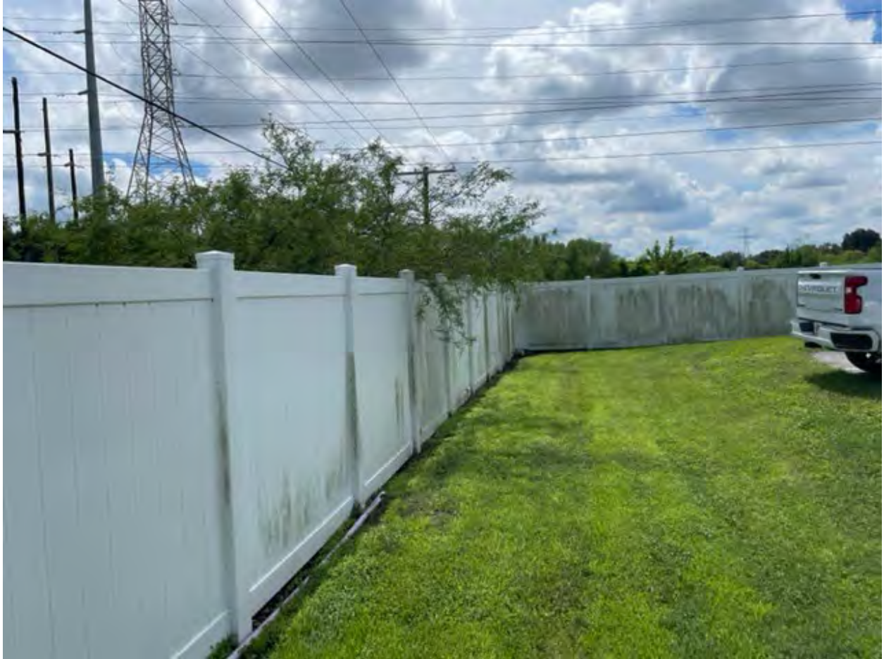
Fence is very dirty in this area, recommend a pressure washing.
