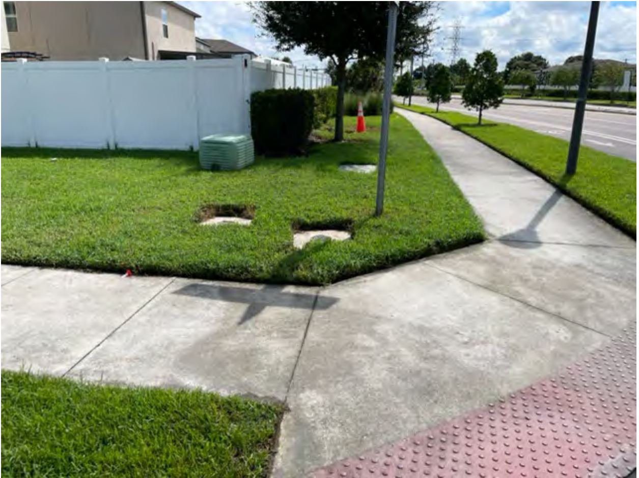
Irrigation leak has been resolved on the corner of Camden Field and Wild Senna.
