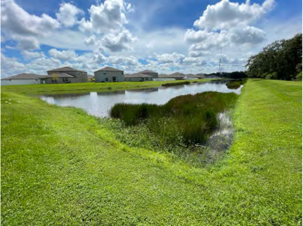
Pond 4 looks good overall, alligator weed is just starting to grow into cattails, should be sprayed at next pond maintenance visit.
