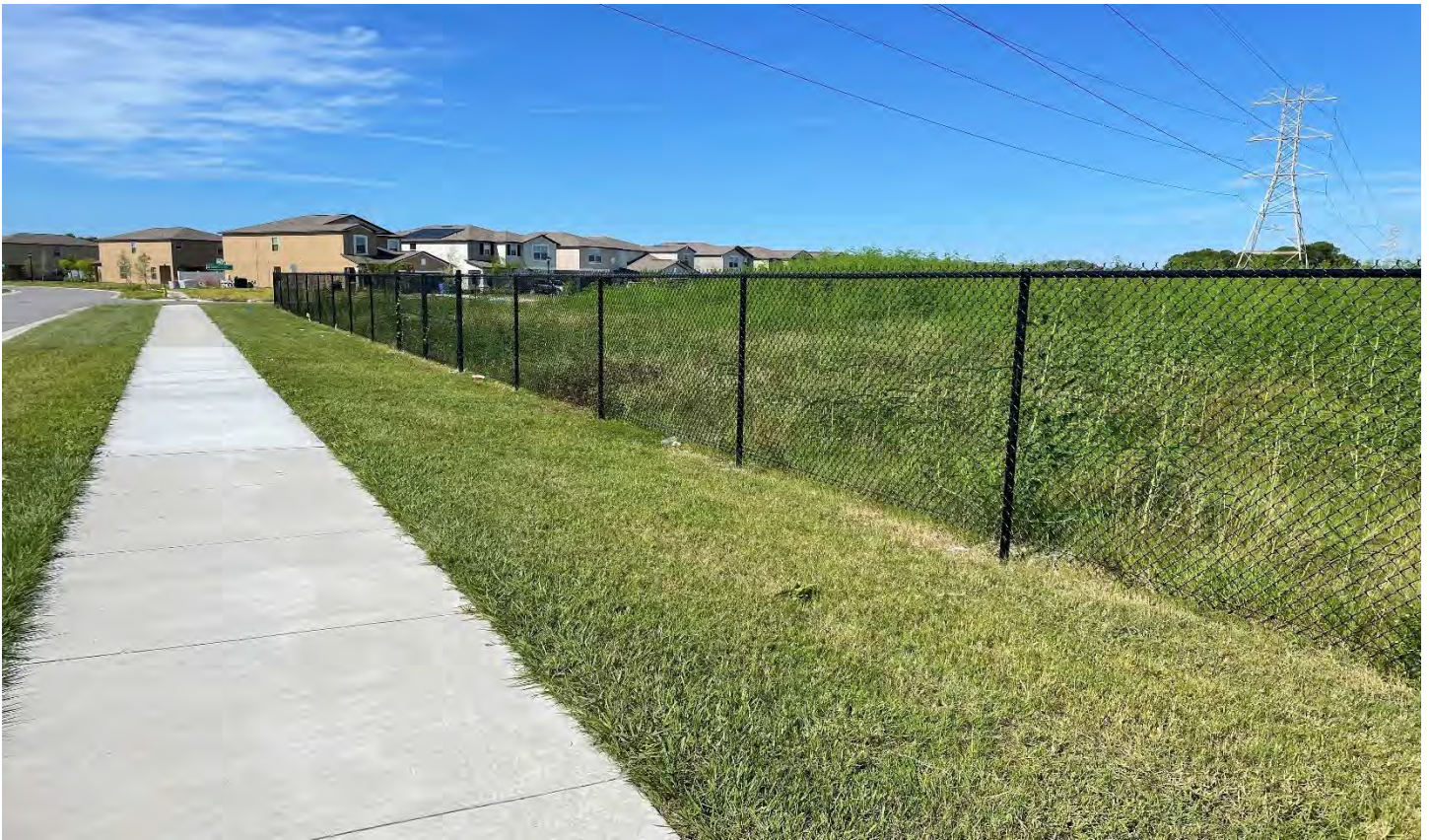
A chain link fence has been installed around the TECO easement. They still have not mowed it despite a written and verbal request.
