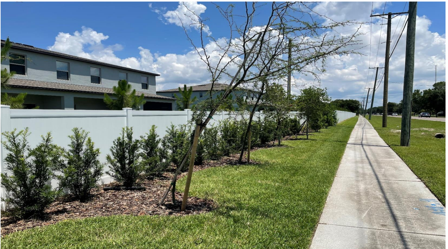
Steadfast is having trouble keeping the trees staked up along 78 th street further North of the entrance where the landscape was turned over not too long ago.
