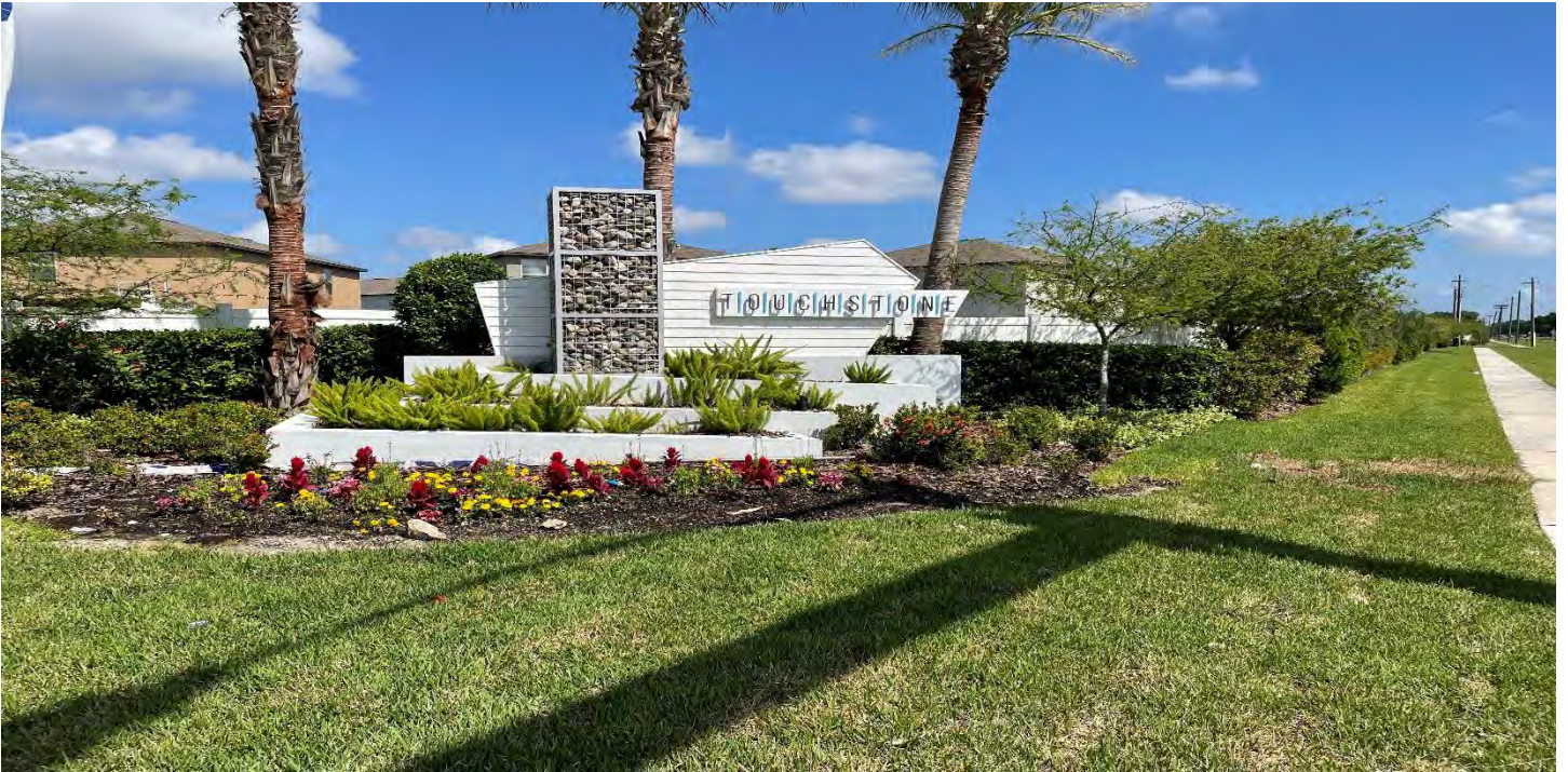
The utility contractors have finished adding the valve at the entrance.
