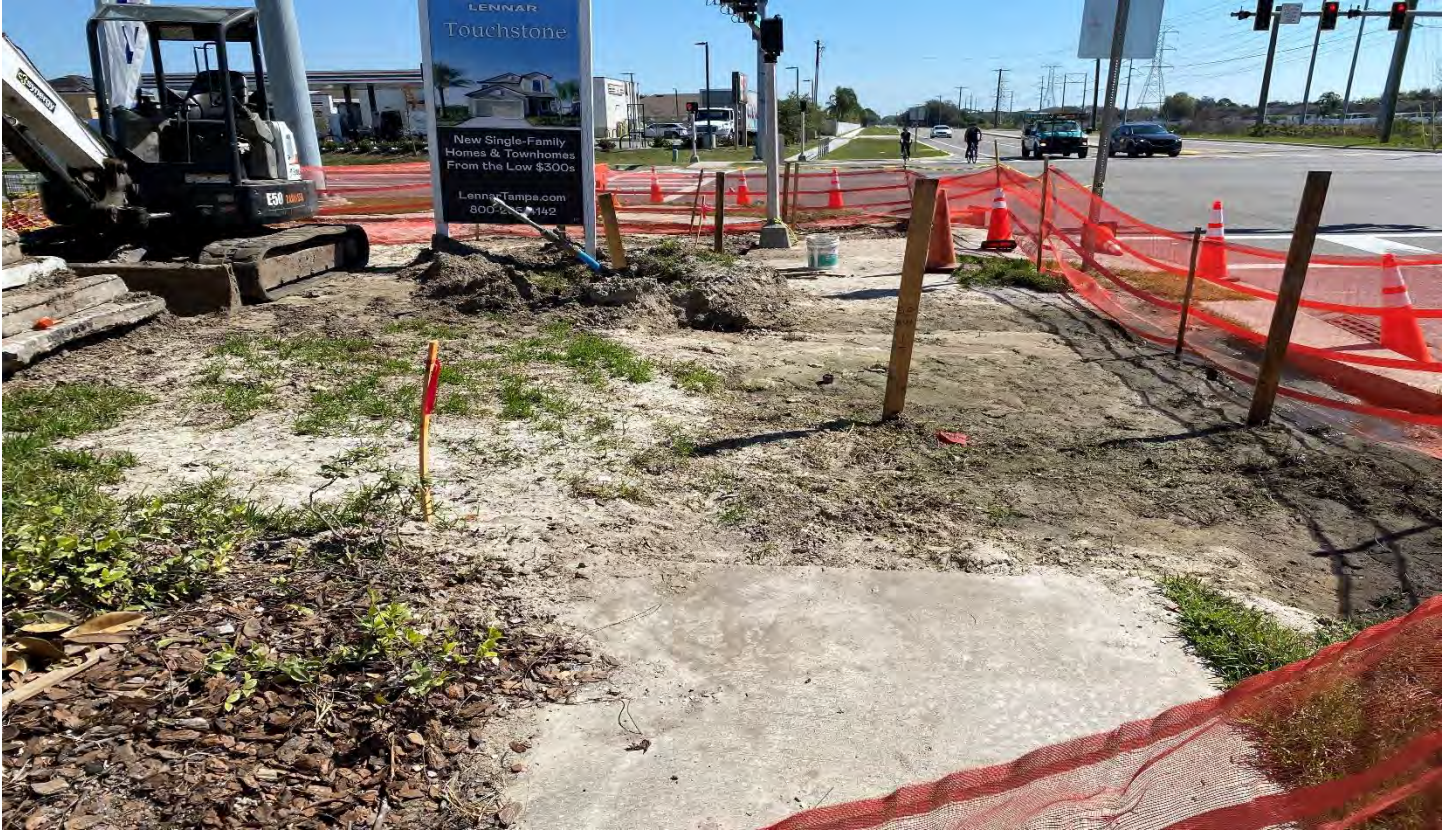
Utility construction is still taking place at the front entrance.
