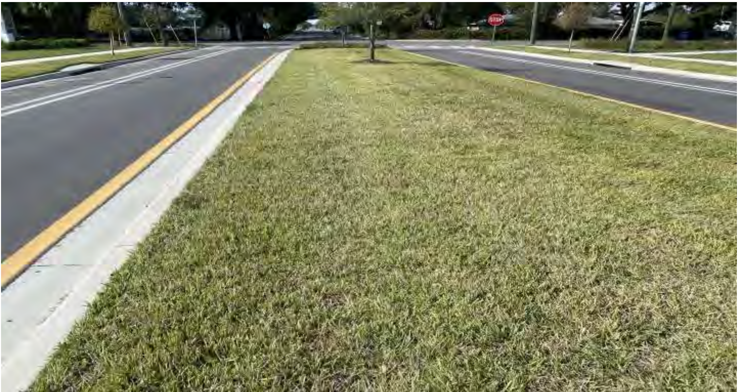
The turf along the Camden Fields extension is in good condition.
