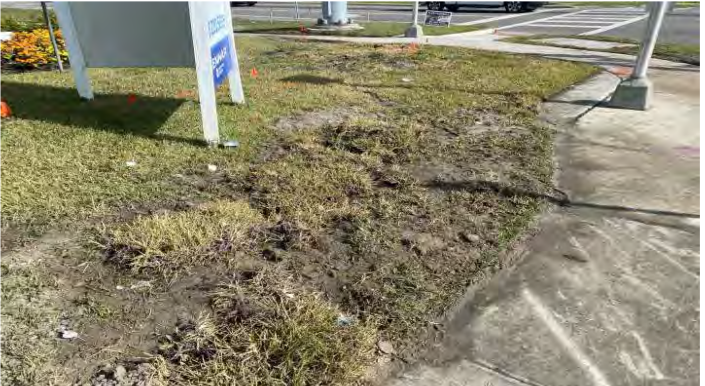
The utility companies have torn up the sod at the entrance.
