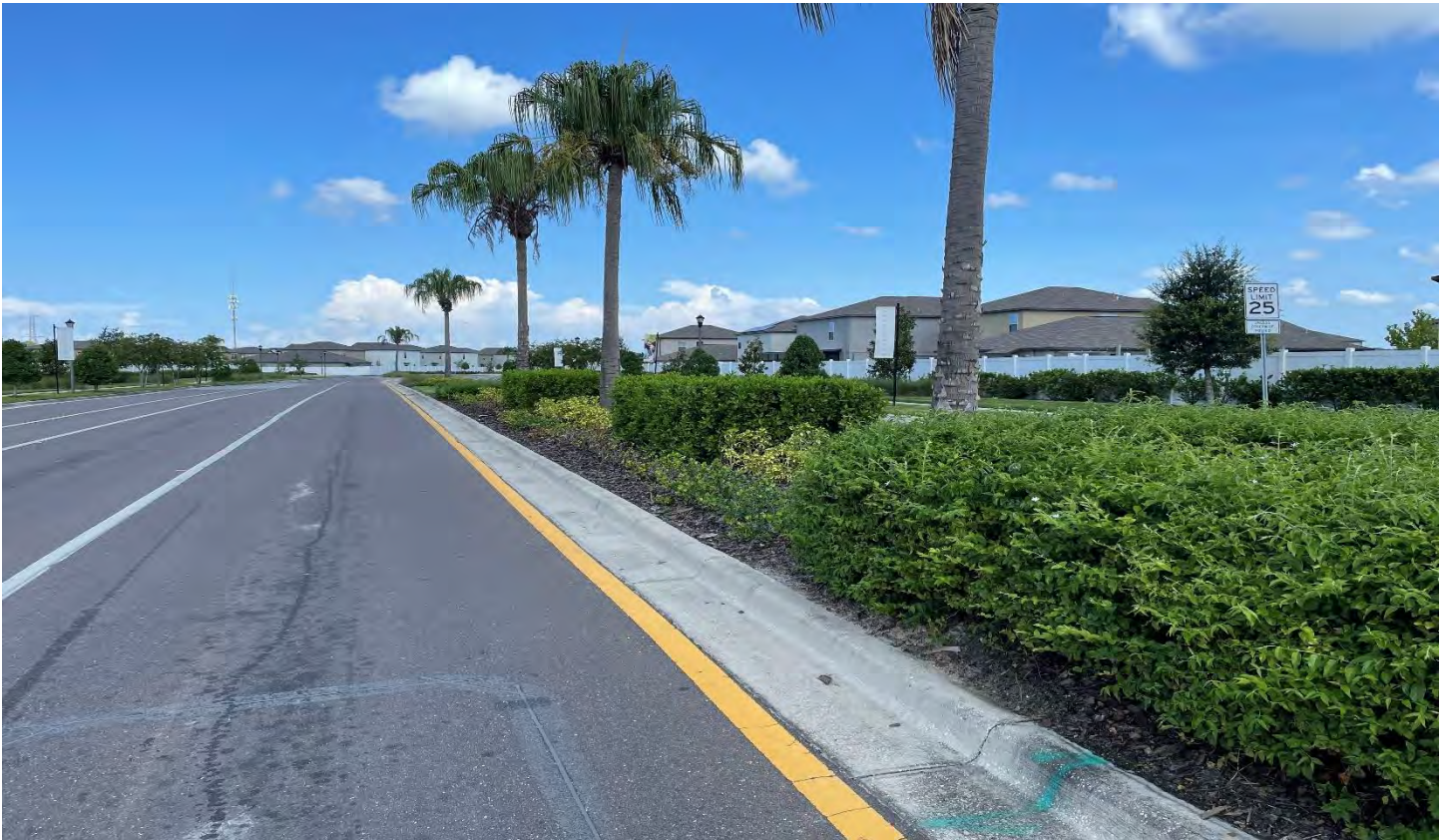
The landscape in the median at the entrance is in good condition.
