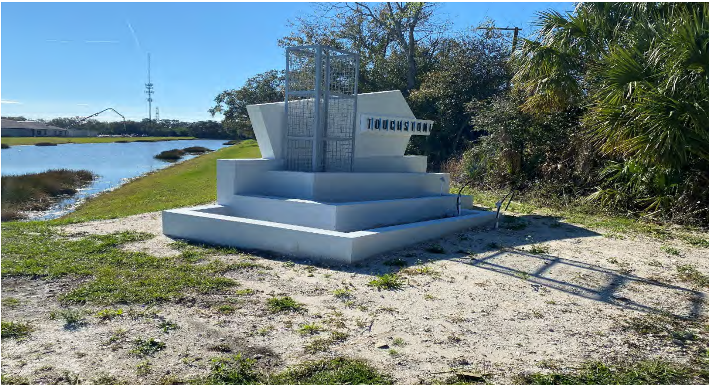
The Touchstone sign at Camden Fields and 70 th street is almost completed.
