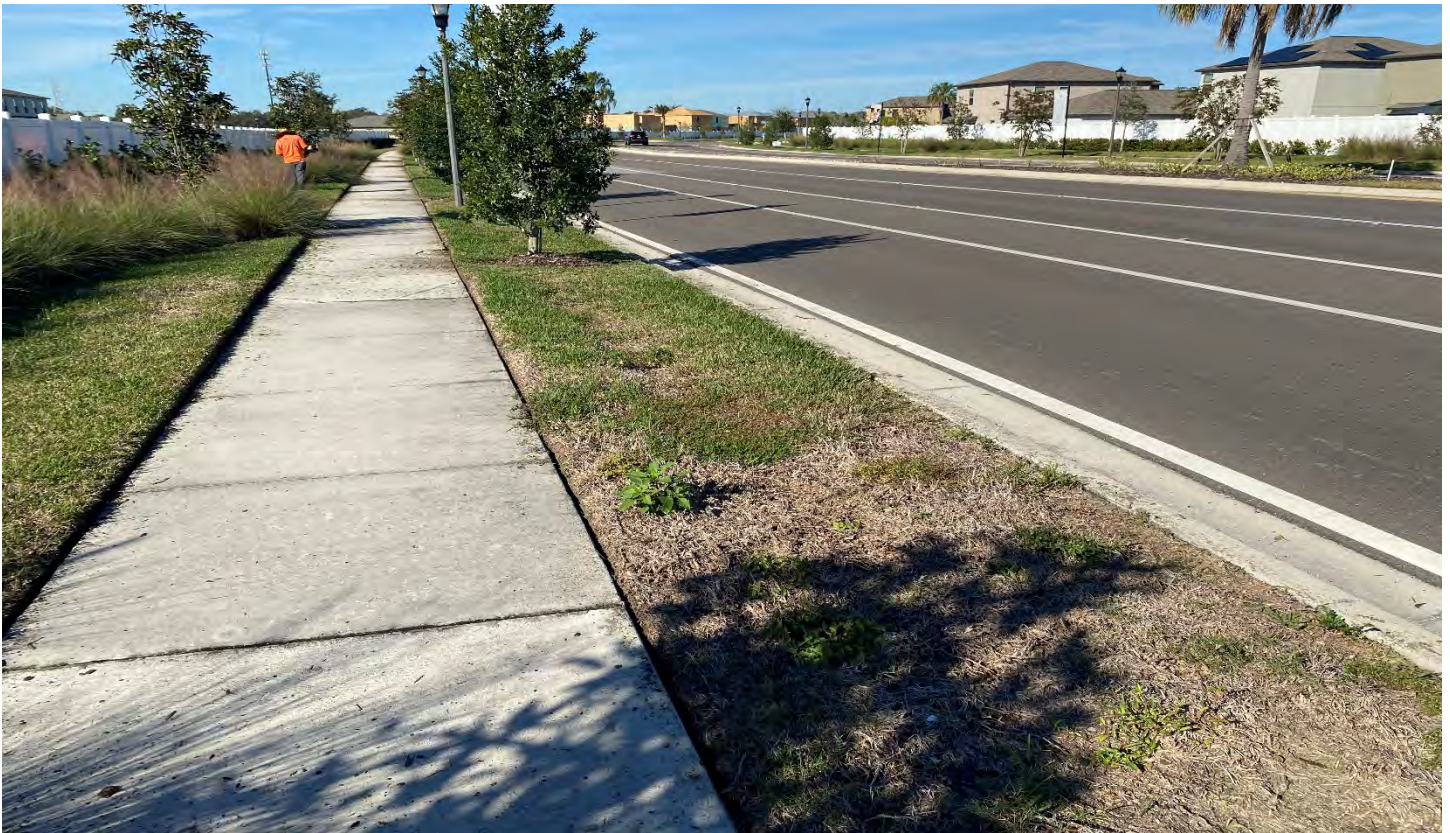
There are several areas of chinch bug damage along Camden Fields.
