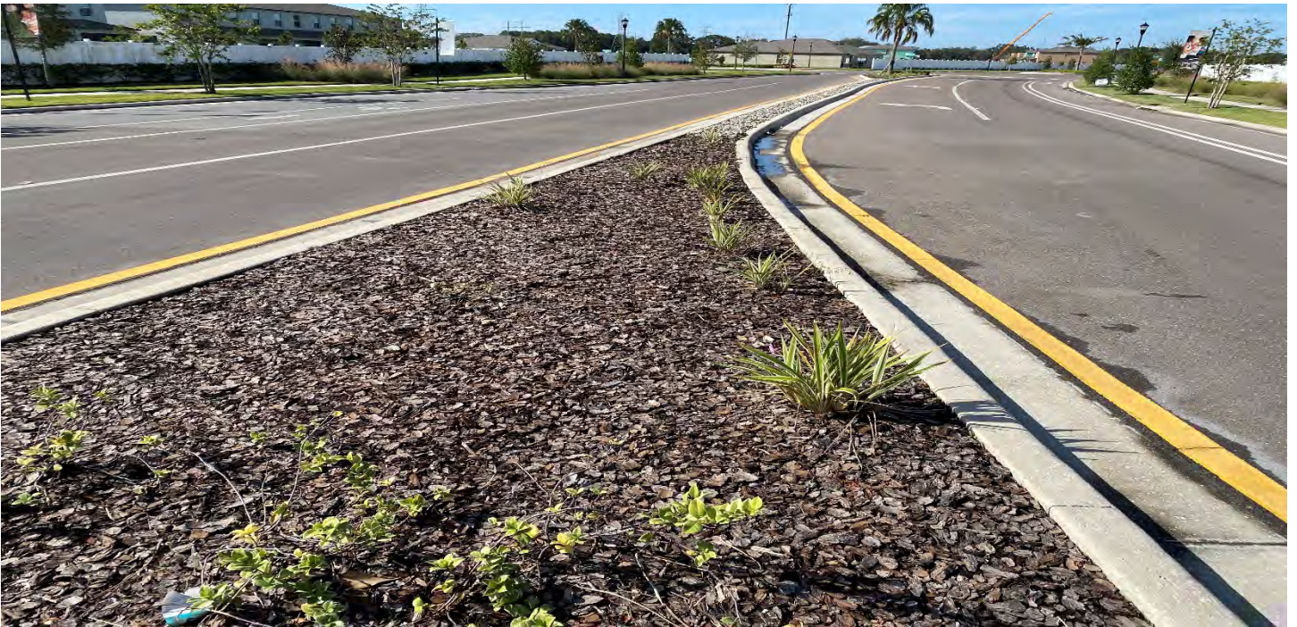
Most of the Flax lilies in the median have died due to the median holding water.
