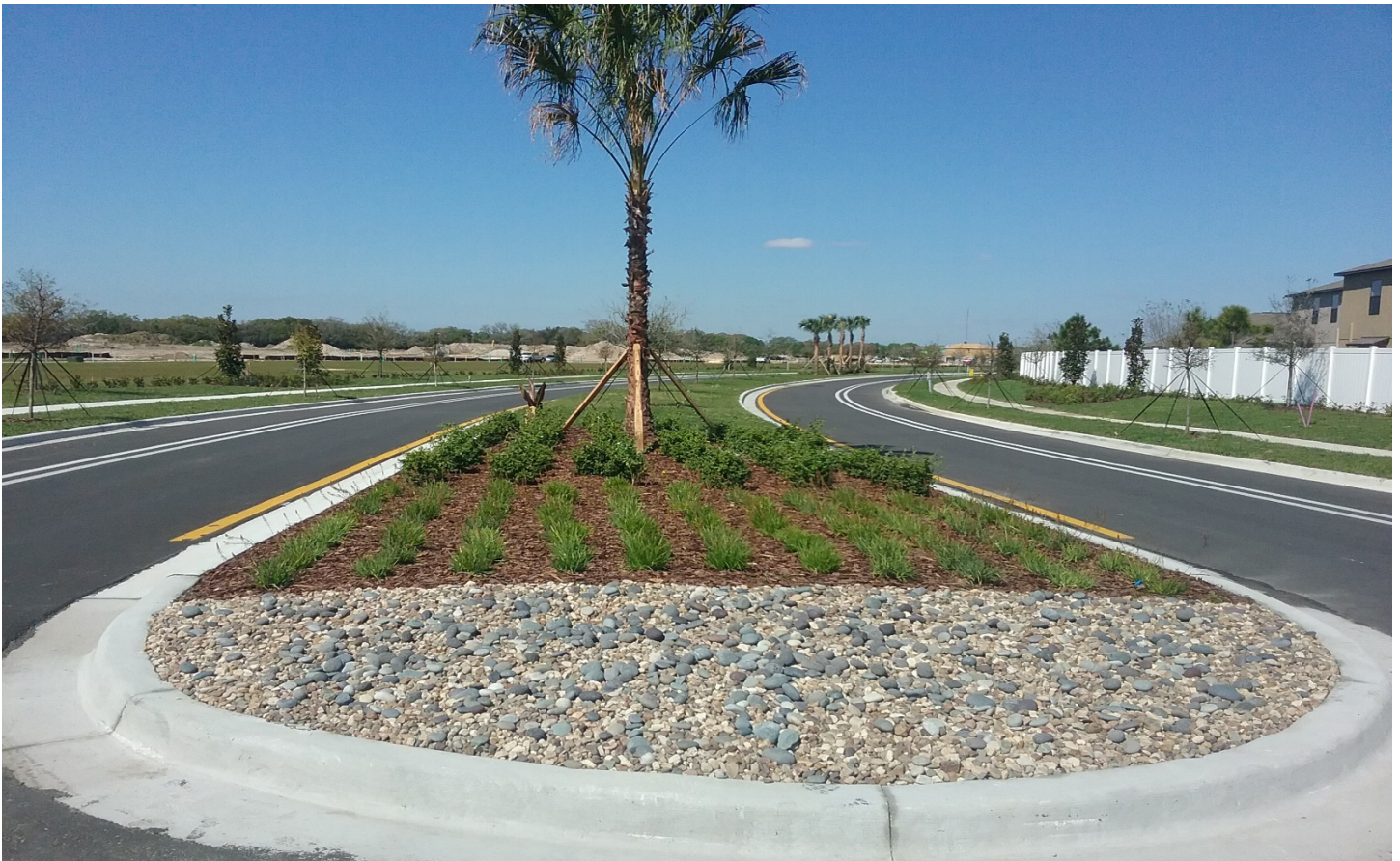
Landscape installation along Camden Field extension has been completed.
