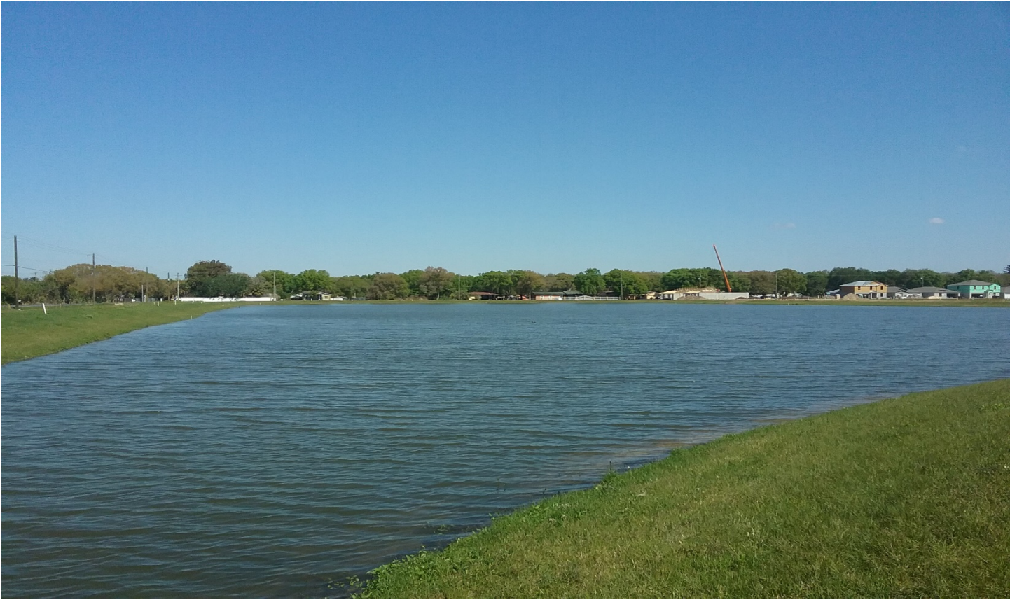
The conditions of pond 3 has improved.
