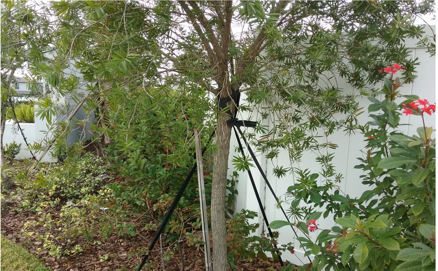
Some of the tree straps are beginning to girdle the trunks and need to be removed.
