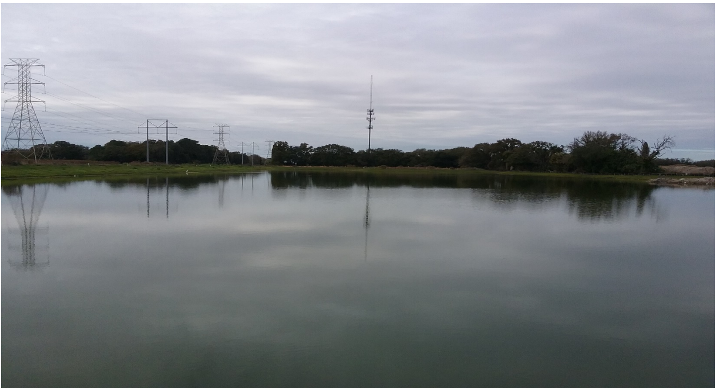
Pond 5 is in good condition.
