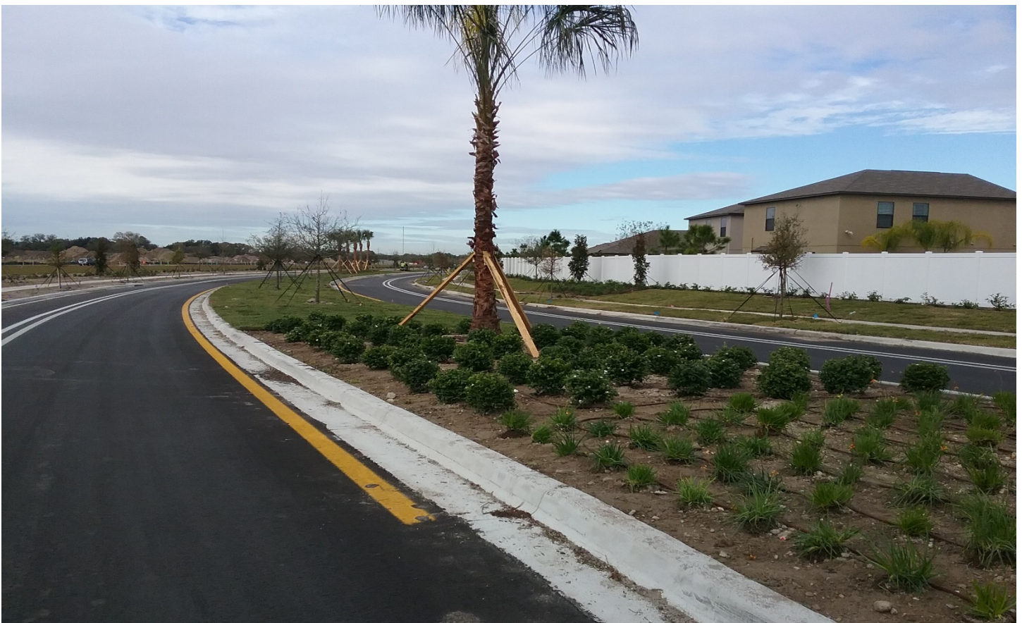
The Camden Fields extension is in the process of being landscaped.
