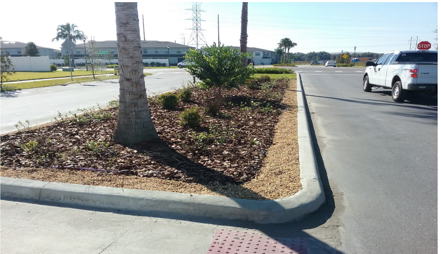
Drains were added to the median on Wild Senna.
