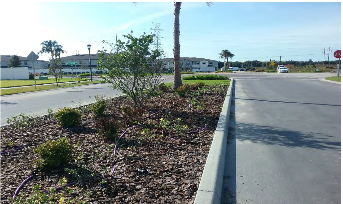
Dead plant material on Wild Senna still needs to be replaced.
