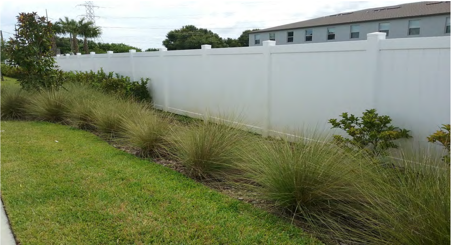
The dead viburnum plants have been removed leaving gaps.
