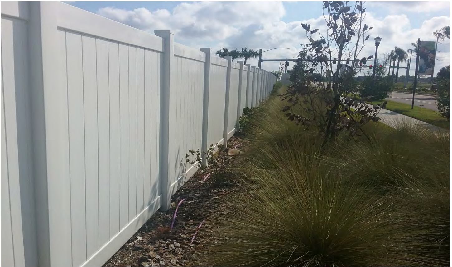
There are voids along the fence where the dead viburnum plants were removed.
